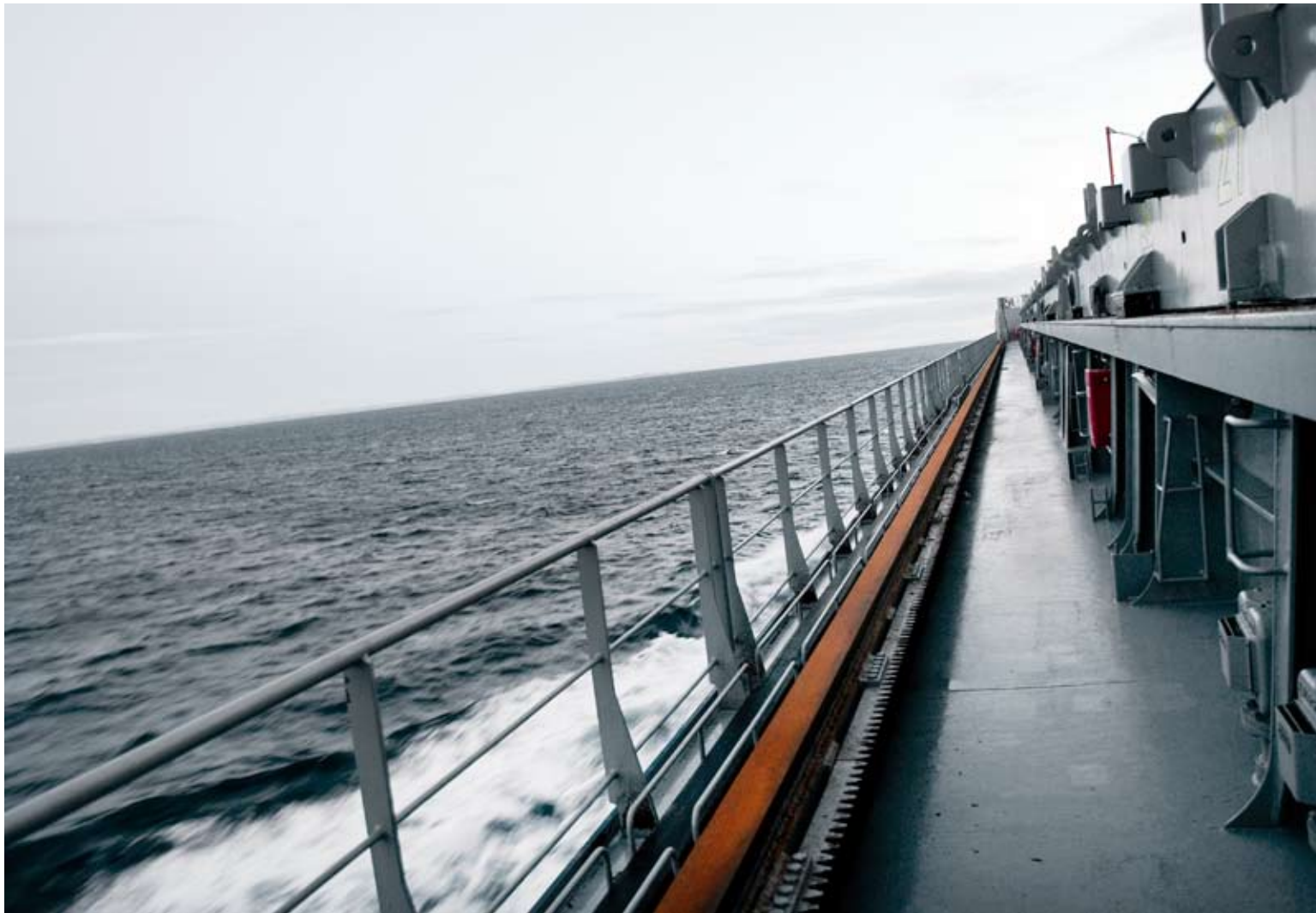
The gantry crane can move 150 metres along the vessel side. The crane gets traction from the Gantry travel rails seen on the picture
